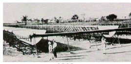
1913 CSP Experimental Plant Built by Frank Shuman (Cairo)
