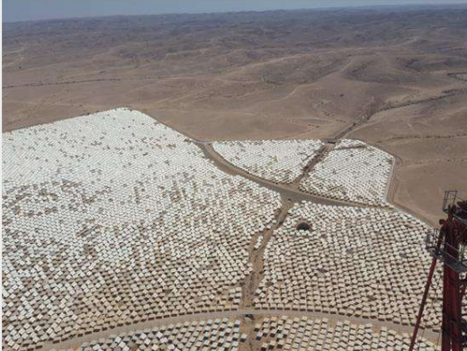
Solar field reflectors
