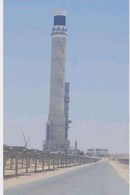
Solar tower receiver
