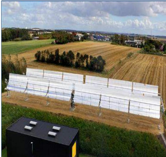
144 m Parabolic shaped mirrors
