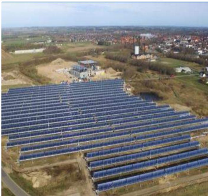
40 rows of 125m parabolic troughs
