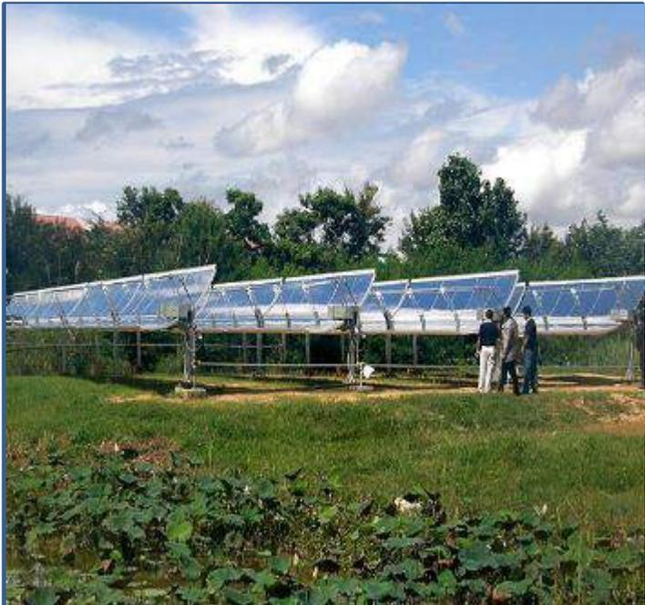
Parabolic trough collectors
